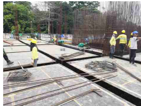
Large span between props to provide wide walk-through area on site
