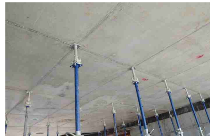
Smooth concrete surface effect after formwork dismantled
