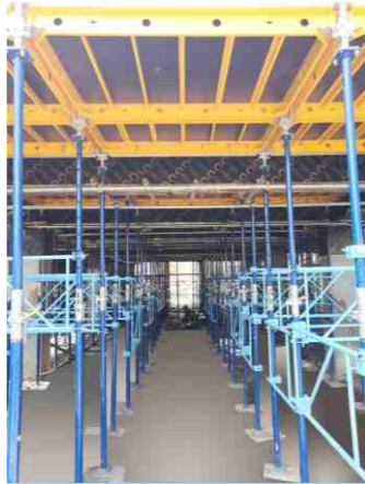
Large span between props to provide wide walk-through area on site
