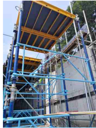
Reinforcement with truss for high shoring support
