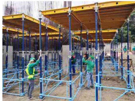
4 workers as one group to assemble and dismantle formwork
