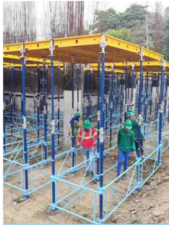
4 workers as one group to assemble and dismantle formwork
