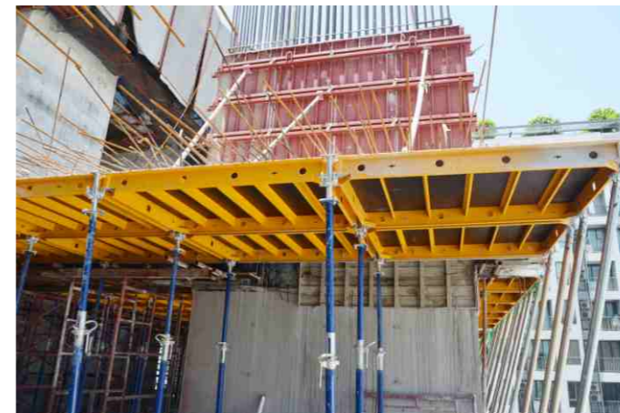
Combine fastform slab formwork with wall formwork for construction
