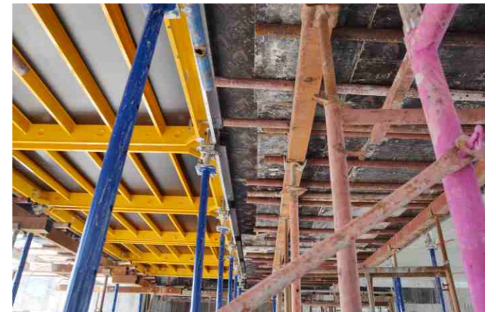
Combine fastform slab formwork with conventional formwork for construction
